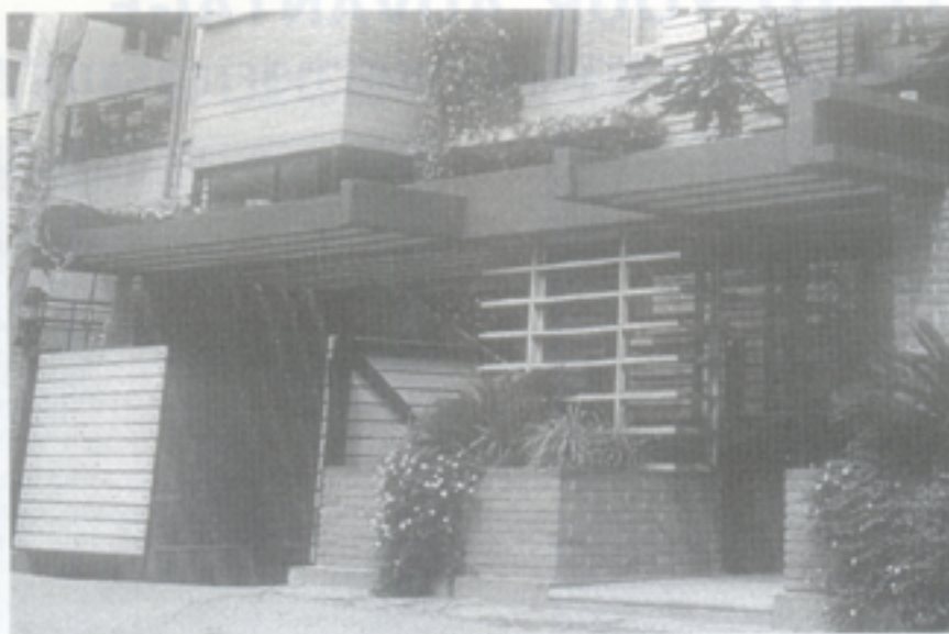
View of the security cabin
